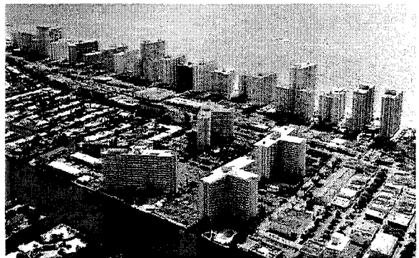
Galt Mile Condominium Association, a 27 building, 6,400 unit association that would be required to retrofit with sprinklers.
