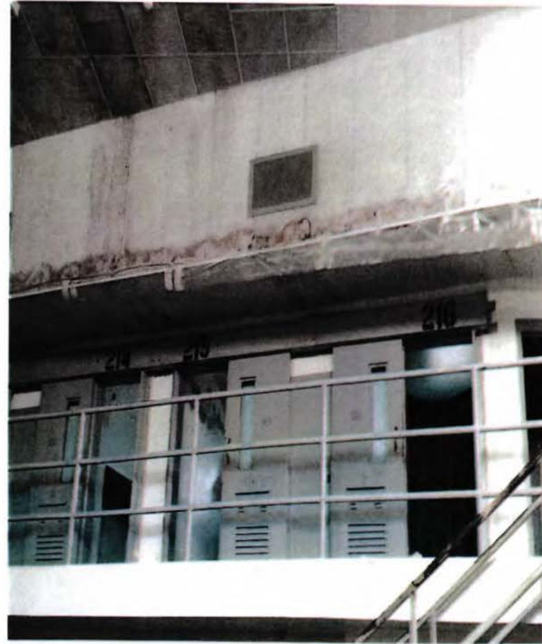
Examples of Leaking Roofs
