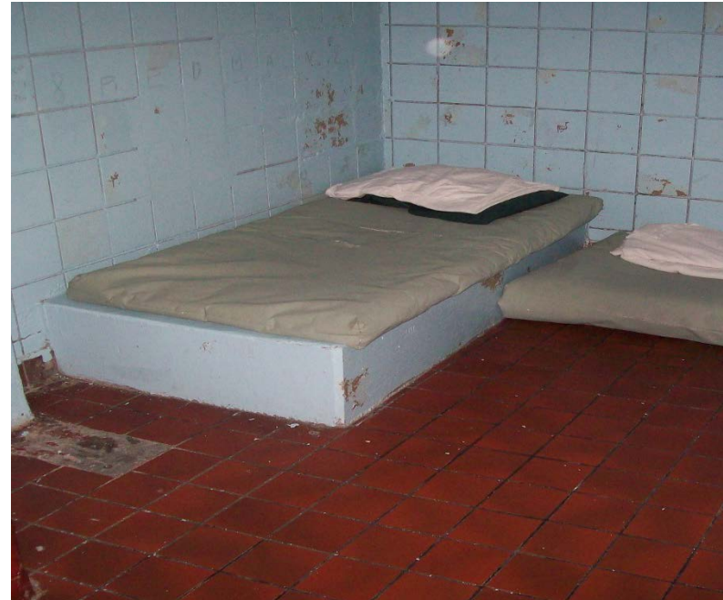
Renovate youths' rooms Hillsborough West Regional Juvenile Detention Center
