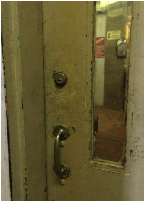
Replace doors and locks Broward Regional Juvenile Detention Center
