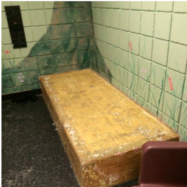
Renovate youths' rooms Broward Regional Juvenile Detention Center
