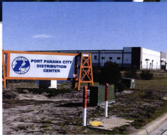
Port Panama City Intermodal Distribution Center
